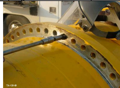
Cleaning paint and rust prior to torquing
