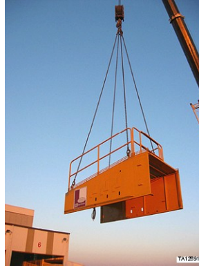
Figure 13: Hoisting of hood assembly
