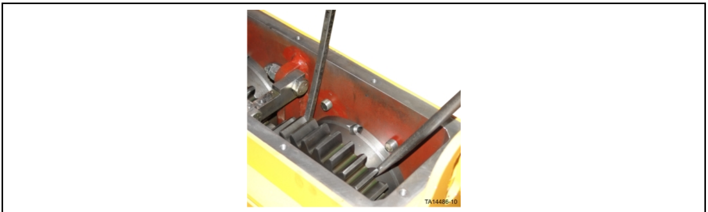
Figure 27: Gear pried toward rear of gearbox
