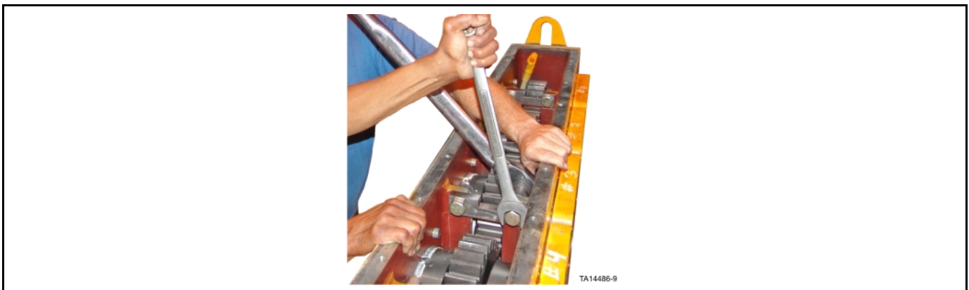
Figure 25: Installation of brace bars
