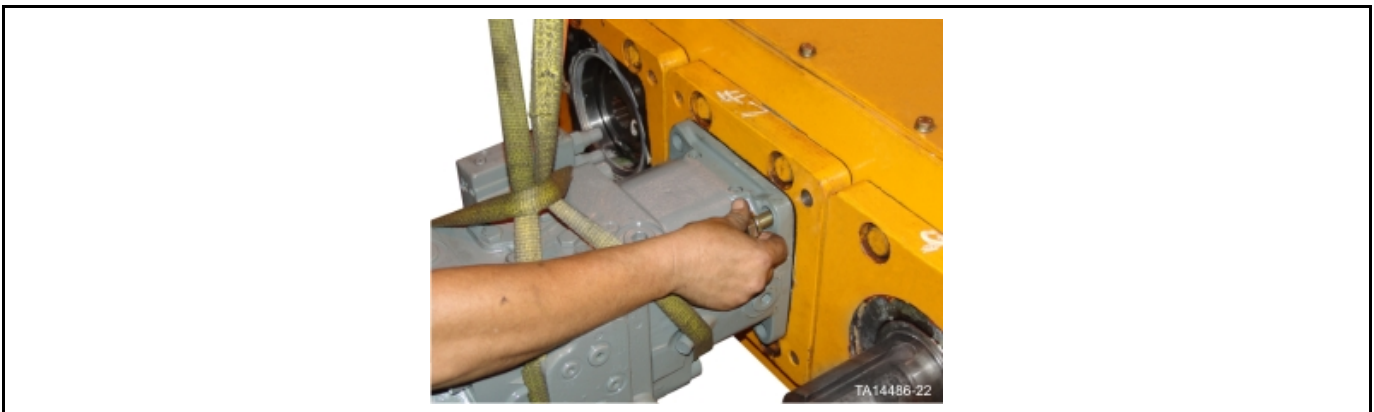
Figure 40: Installation of pumps retaining bolts & flat washers
